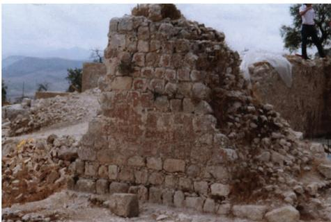
Fig. 8. Ruins of the Castle of Cañete la Real (Malaga, Spain). The piece of wall shows extensive loss of joint mortar linking the stone blocks.
