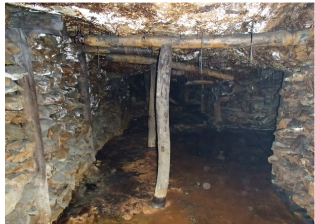
Fig 7. Old adit with rock wall made of waste. (Source: photography from the authors).
