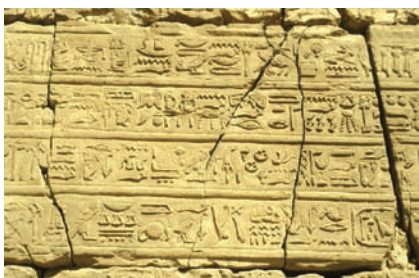
fig 10. Fissures, Karnak Temple / Luxor (Egypt).
